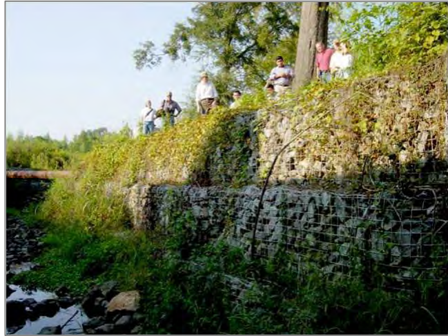
Figure 1: Retaining wall made of gabions
