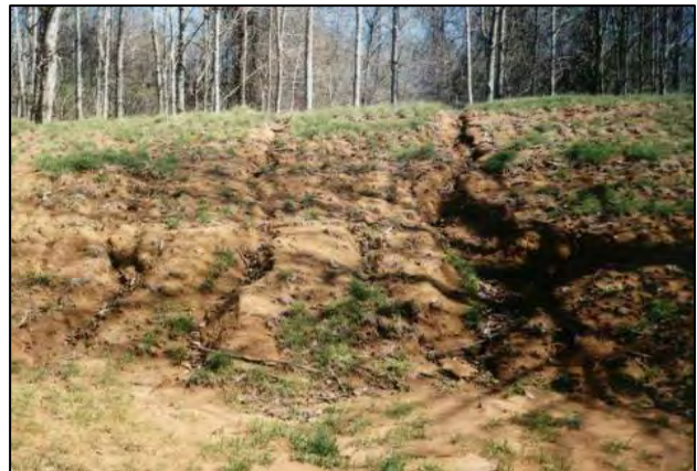
Figure 3 Rill Erosion
