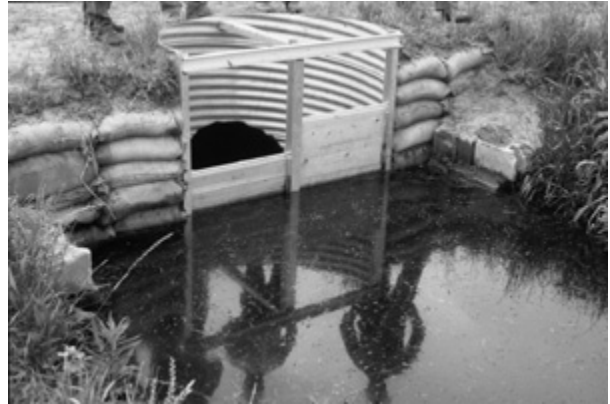
Flashboard Riser (Source: NRCS)
