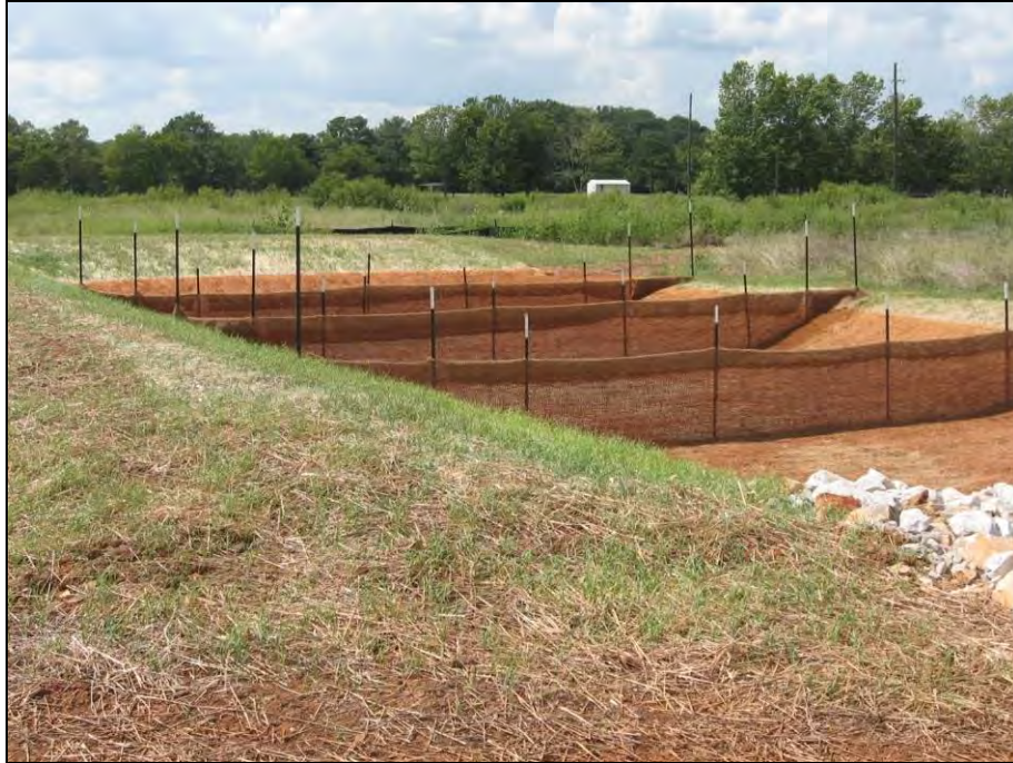
Figure SBN-3 Example of porous baffle made of 700 g/m 2 coir erosion blanket as viewed from the inlet
