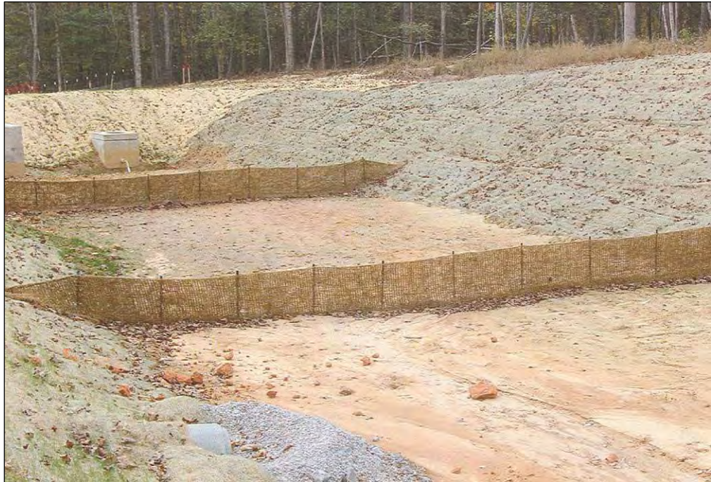
Figure SBN-2 Example of porous baffle made of 700-g/m 2 coir erosion blanket as viewed from the inlet (Source: North Carolina Erosion and Sediment Control Planning and Design Manual)
