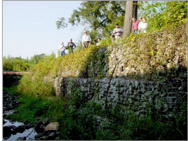
Figure 1: Retaining wall made of gabions
