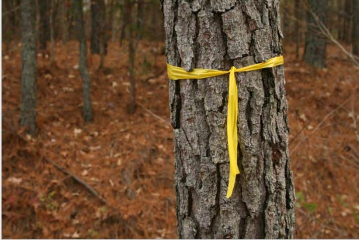
Limits of clearing should be planned outside the drip line of groups or individual trees to be saved. The clearing should never be closer than 5 feet to the trunk of a tree.
