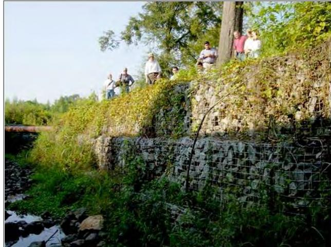
Figure 1: Retaining wall made of gabions
