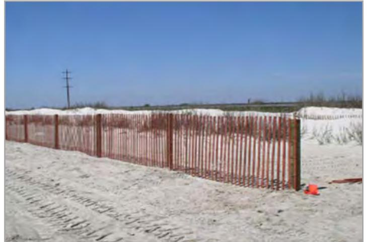
Figure 1 Sand Fence (<http://www.gulfmex.org/crp/7004/fence.jpg>)
