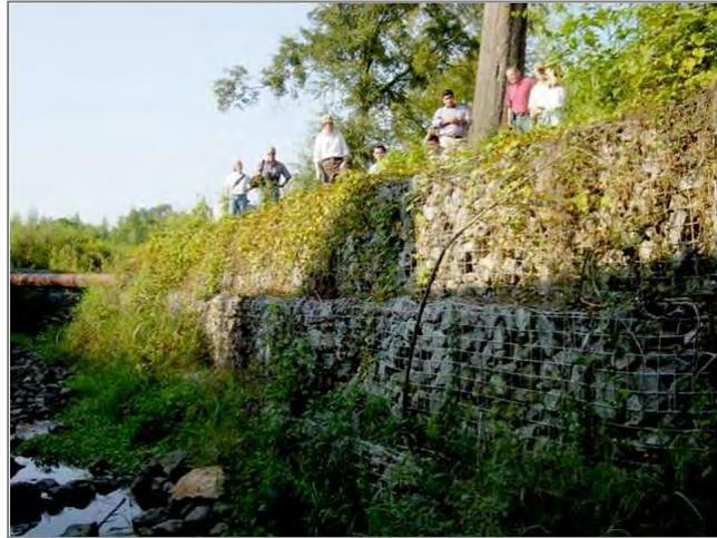
Figure 1: Retaining wall made of gabions
