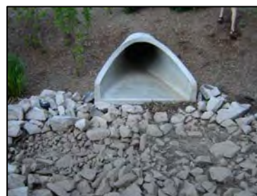
Figure 3 Bioretention Cell with Pretreatment Forebay
