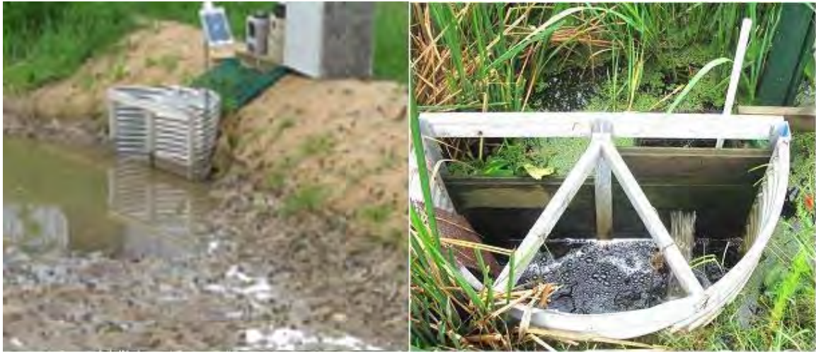
Figure 4 Outlet Structure with Flashboard Riser for Maintenance (Photos Courtesy of NC State Science House & BAE)
