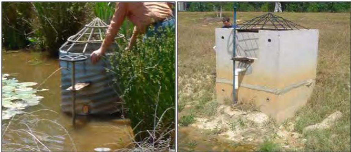
Figure 3 Outlet Structures with Manual Drawdown Valve for Maintenance
