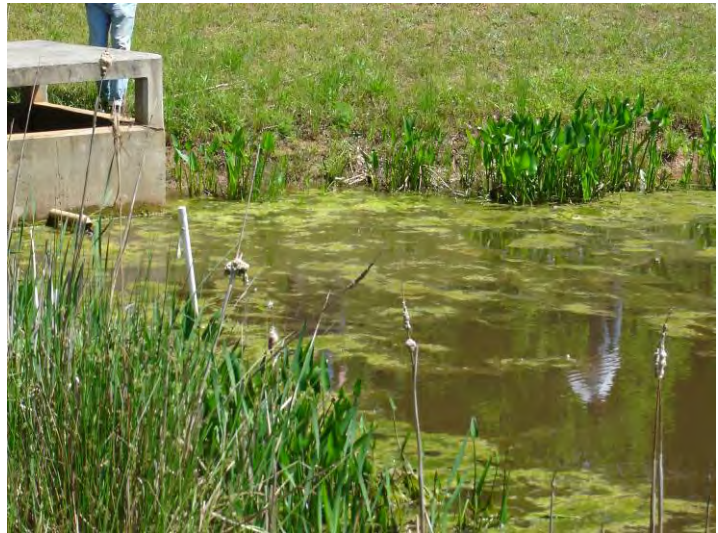
Figure 4 Outlet Structure Near Wetland Edge, Orifice Easily Accessible for Maintenance
