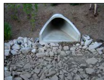
Figure 3 Bioretention Cell with Pretreatment Forebay
