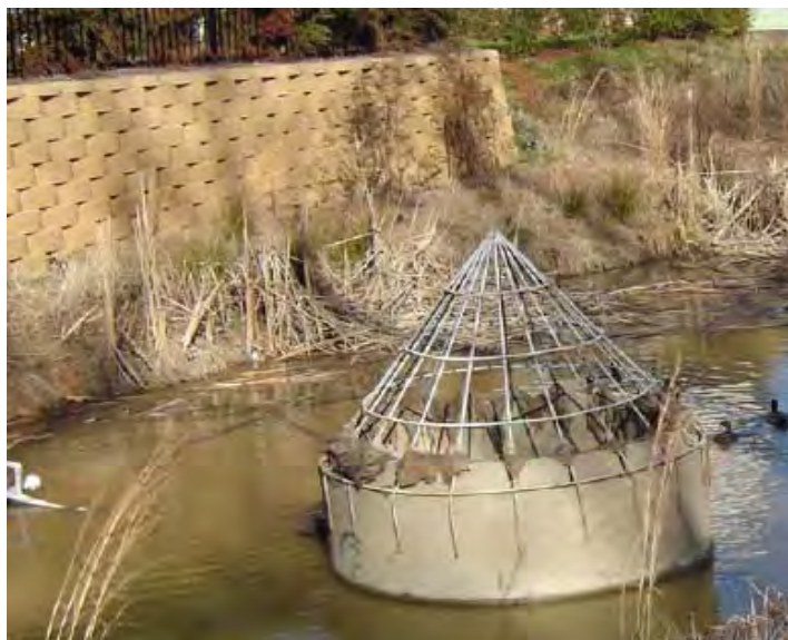
Figure 5 Outlet Structure Not Near Wetland Edge, Orifice Not Easily Accessible for Maintenance
