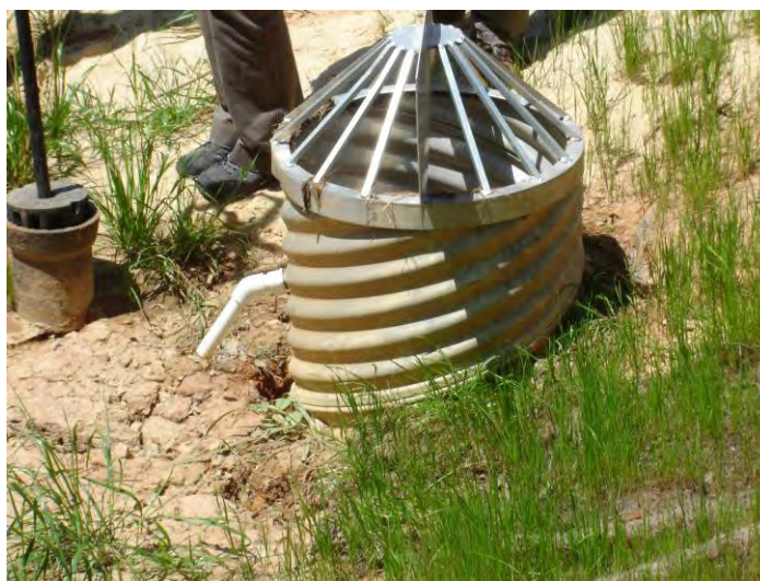
Figure 5 Outlet Structure with Down-Turned Drawdown Orifice
