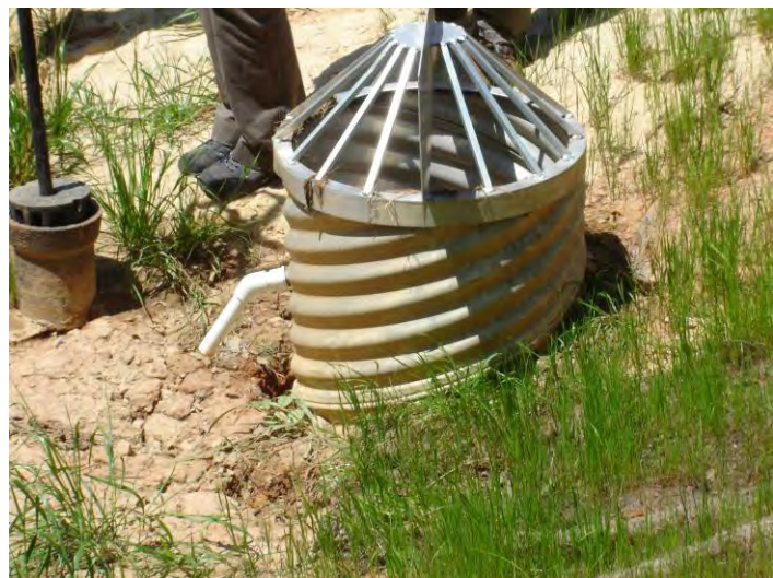
Figure 5 Outlet Structure with Down-Turned Drawdown Orifice
