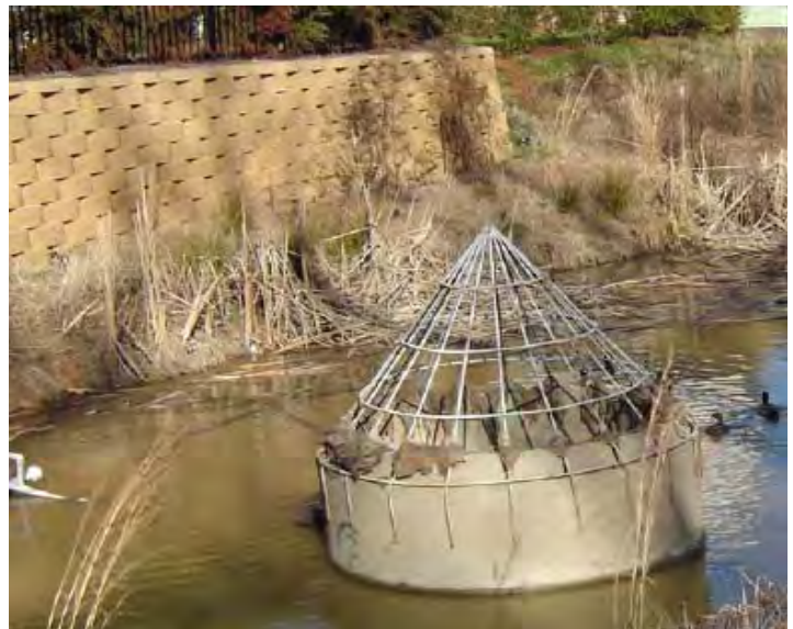
Figure 5 Outlet Structure Not Near Wetland Edge, Orifice Not Easily Accessible for Maintenance
