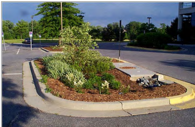
Figure 1 Bioretention in Parking Lot Island
