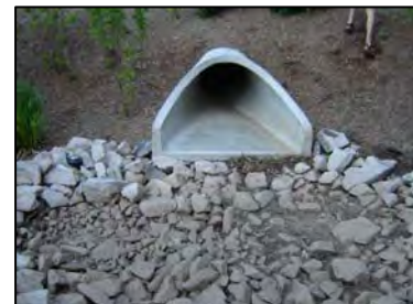
Figure 3 Bioretention Cell with Pretreatment Forebay
