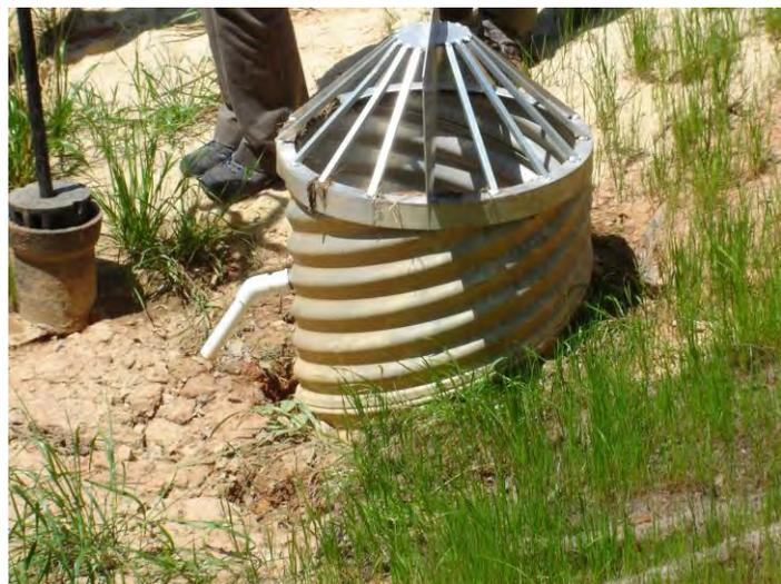
**Figure 5 Outlet Structure with Down-Turned Drawdown Orifice**
