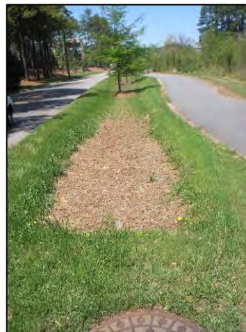
Figure 2 Bioretention Cell with Pretreatment: Gravel and Grass (Needs Maintenance)
