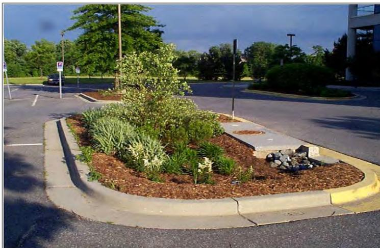
Figure 1 Bioretention in Parking Lot Island
