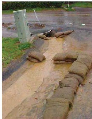
Figure 5. Make sure storm drain inlets are protected.
