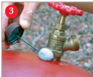
When the spigot is in about halfway, apply a liberal amount of PVC cement to the exposed threads. Continue to screw in the spigot until it is snug and pointing toward the bottom of the barrel.
