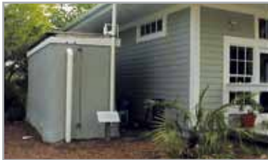
These cisterns at the Florida House Learning Center each hold 2,500 gallons of rainwater.
