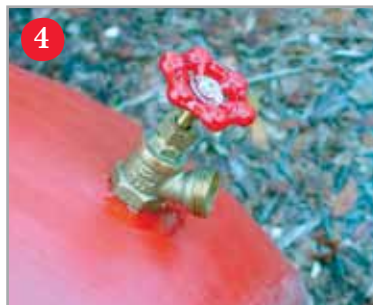
The rain barrel outlet is now complete.
