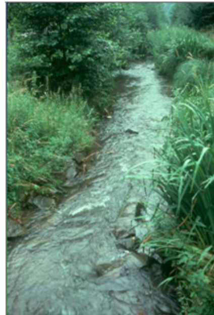
Figure SP-4 Same stream, after bioengineered restoration. This type of bioengineered stream improves habitat, water quality, and numerous other functions that cannot be achieved with hardened stream channels.
