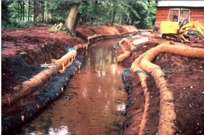
Figure SP-3 Retrofitted urban stream using a bioengineered approach. Note hard, encapsulated-rock toe in lower zone and then coir geotextile rolls to be planted with wetland plants in upper-bank zones.
