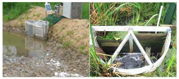
Figure 4 Outlet Structure with Flashboard Riser for Maintenance (Photos Courtesy of NC State Science House & BAE)
