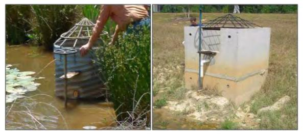
Figure 3 Outlet Structures with Manual Drawdown Valve for Maintenance
