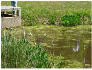
The overflow structure should be located near the edge of the wetland so that it can be accessed easily for maintenance, as shown in Figure 6.
