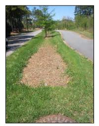
Figure 3 shows a bioretention cell with a pretreatment forebay. Notice the sediment that has settled onto the rocks. Without the forebay, this sediment would have collected on the
