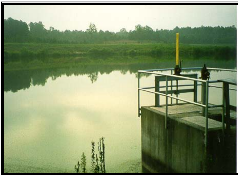
Photo 4. Iuka POTW Facility, Second Cell
