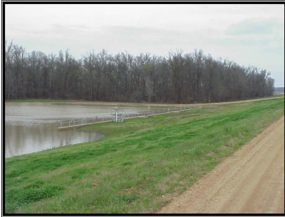
Photo 1. Wasp Lake Upstream of Control Structure
