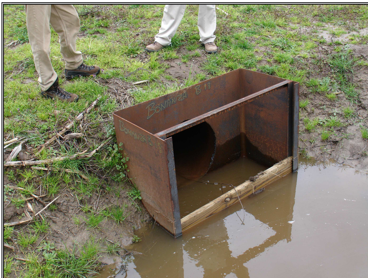
Figure 3. Slotted Board Riser installed on unnamed tributary to oxbow lake in Mississippi Delta
