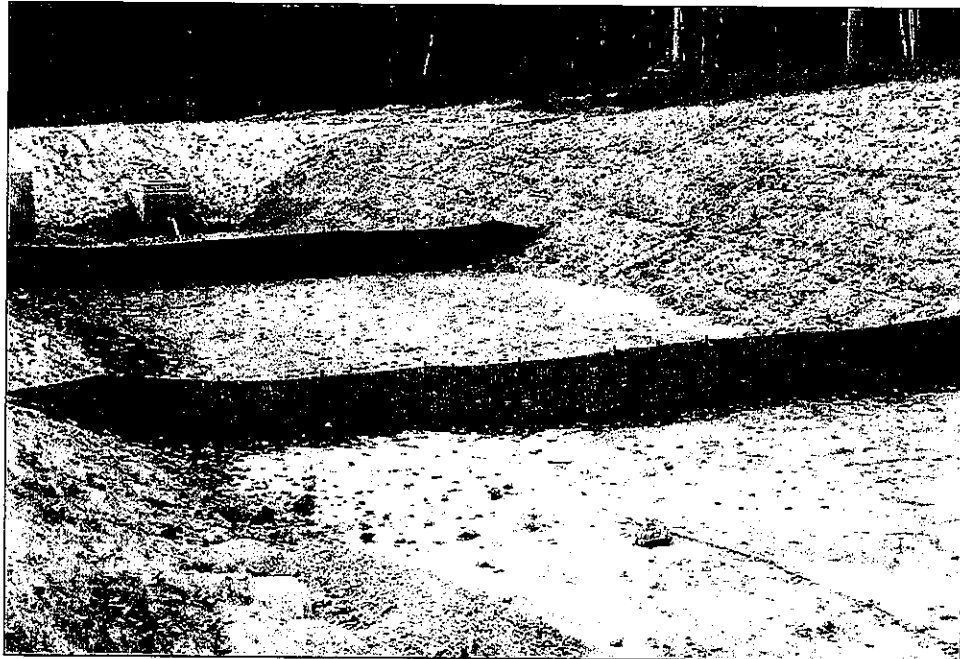
Figure SBN-2 Example of porous baffle made of 700\text{-g/m}^2 coir erosion blanket as viewed from the inlet (Source: North Carolina Erosion and Sediment Control Planning and Design Manual)
