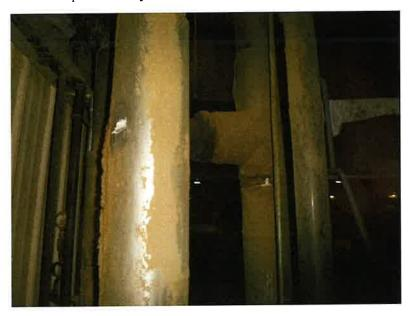
• Gray/Black Pipe Insulation, Fill from Chemical (RB-16 through RB-17). The gray/black pipe insulation is located on the fill from chemical lines and contains 45 percent amosite asbestos and 30 percent chrysotile asbestos.
