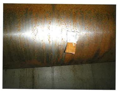
• Brown Pipe Insulation, Chemical (RB-07 through RB-08). The pipe insulation is located on the chemical lines and contains 50 percent amosite asbestos and 10 percent chrysotile asbestos.
