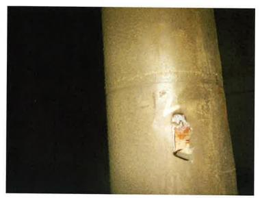
• White Pipe Insulation, Evaporation Pit (RB-23 through RB-25). The white pipe insulation is located near the evaporation pit and contains 50 percent amosite asbestos and 15 percent chrysotile asbestos.
