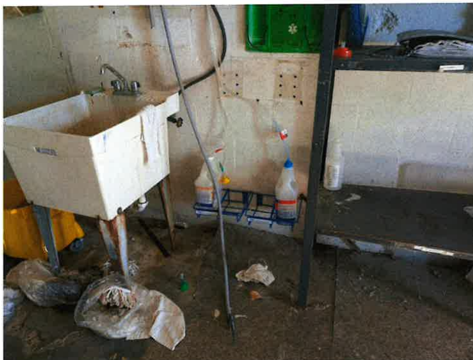
Photo 5: Asbestos-containing sheet vinyl flooring and soap containers in laundry room
