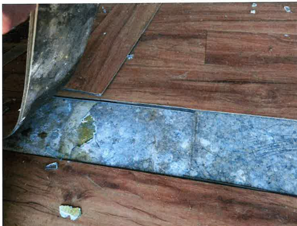
Photo 6: Asbestos-containing sheet vinyl flooring under plank vinyl flooring in Room 128
