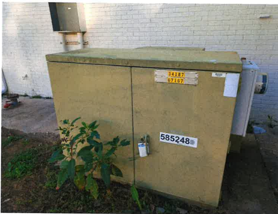
Photo 7: Pad-mounted transformer on north side of building
