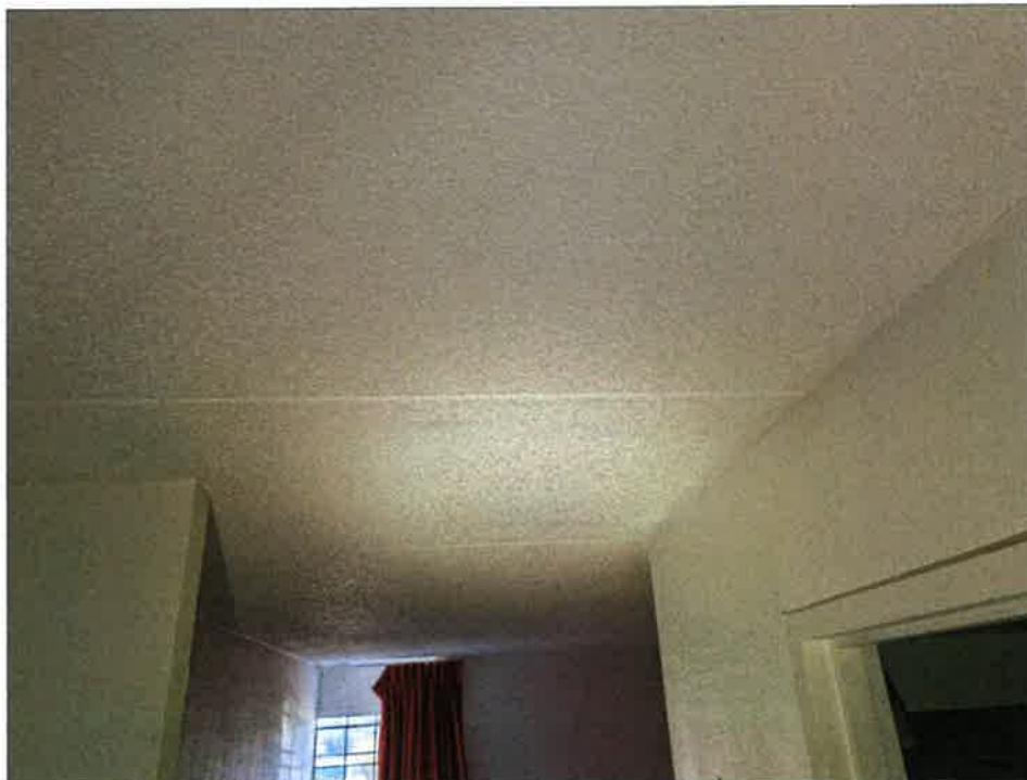
Photo 2: Asbestos-containing spray-applied ceiling texture
