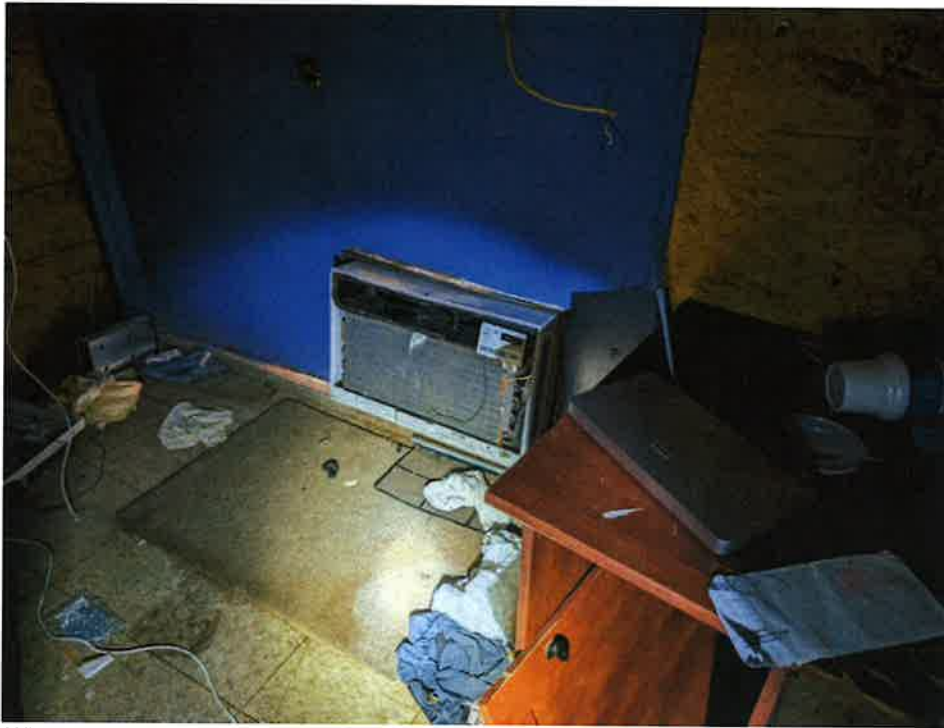
Photo 19: Window HVAC unit in communications room
