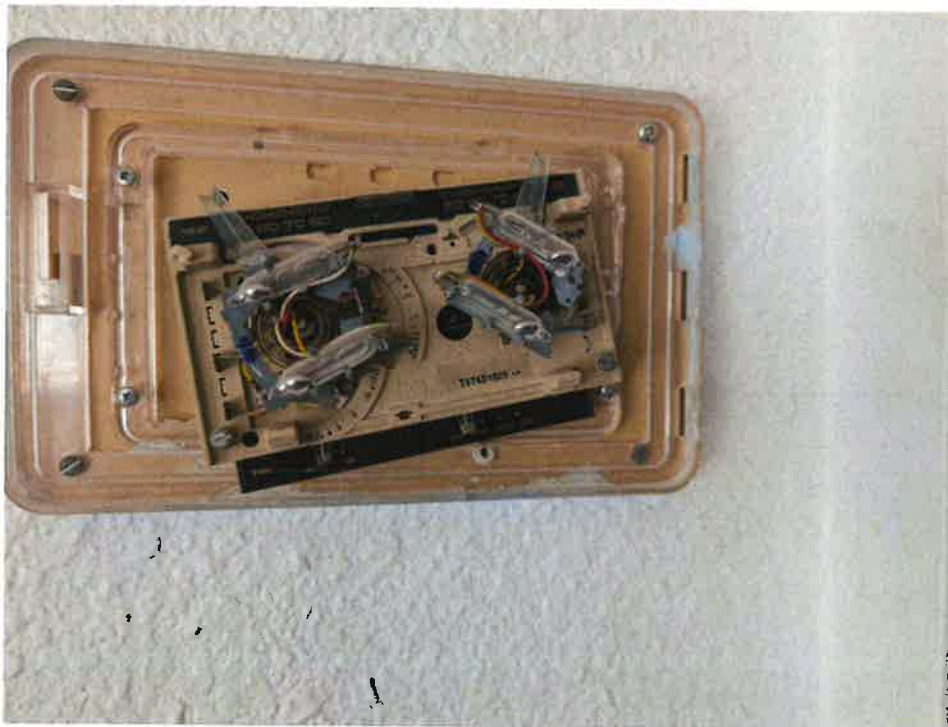
Photo 16: Mercury containing thermostat in banquet hall
