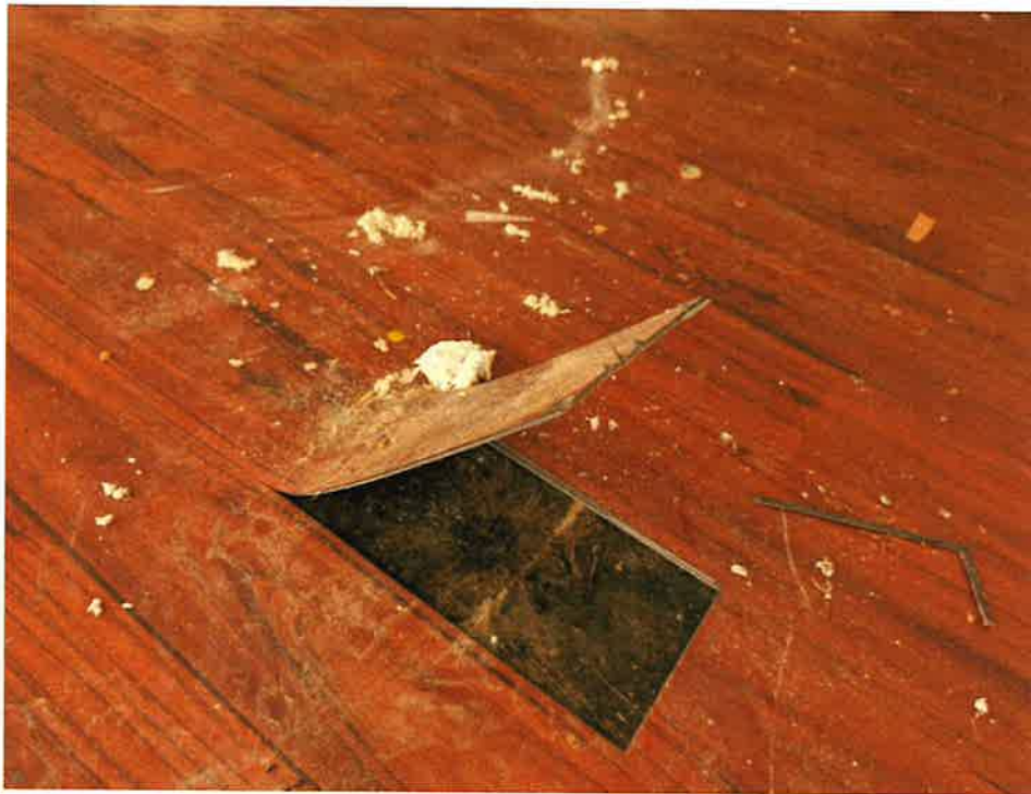
Photo 3: Asbestos-containing black mastic below banquet hall flooring
