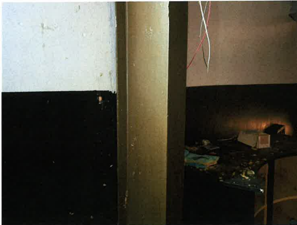
Photo 2: LBP on steel beam
