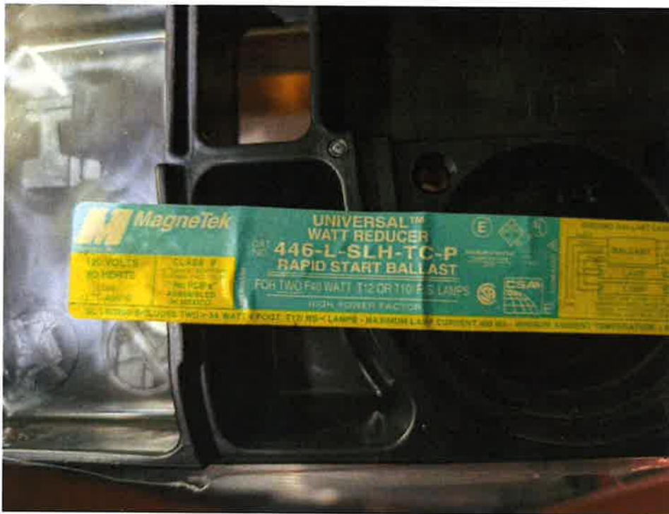
Photo 11: Fluorescent ballast labelled as non-PCB
