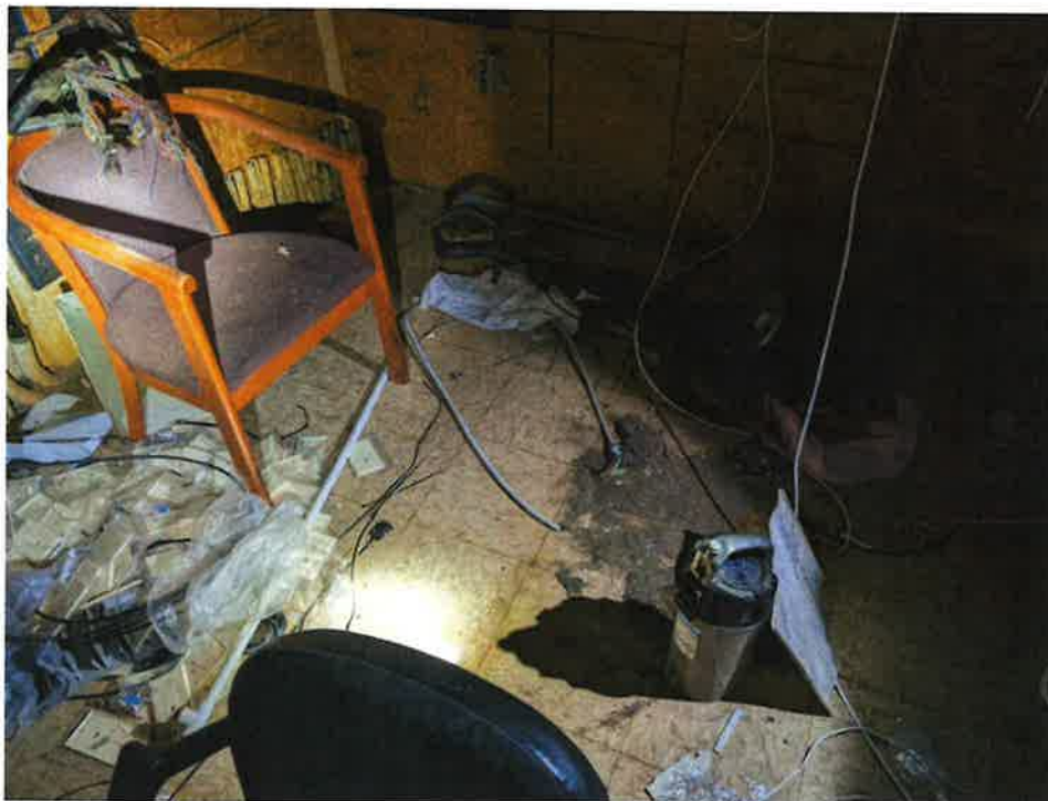
Photo 4: Asbestos-containing black mastic below communications room flooring
