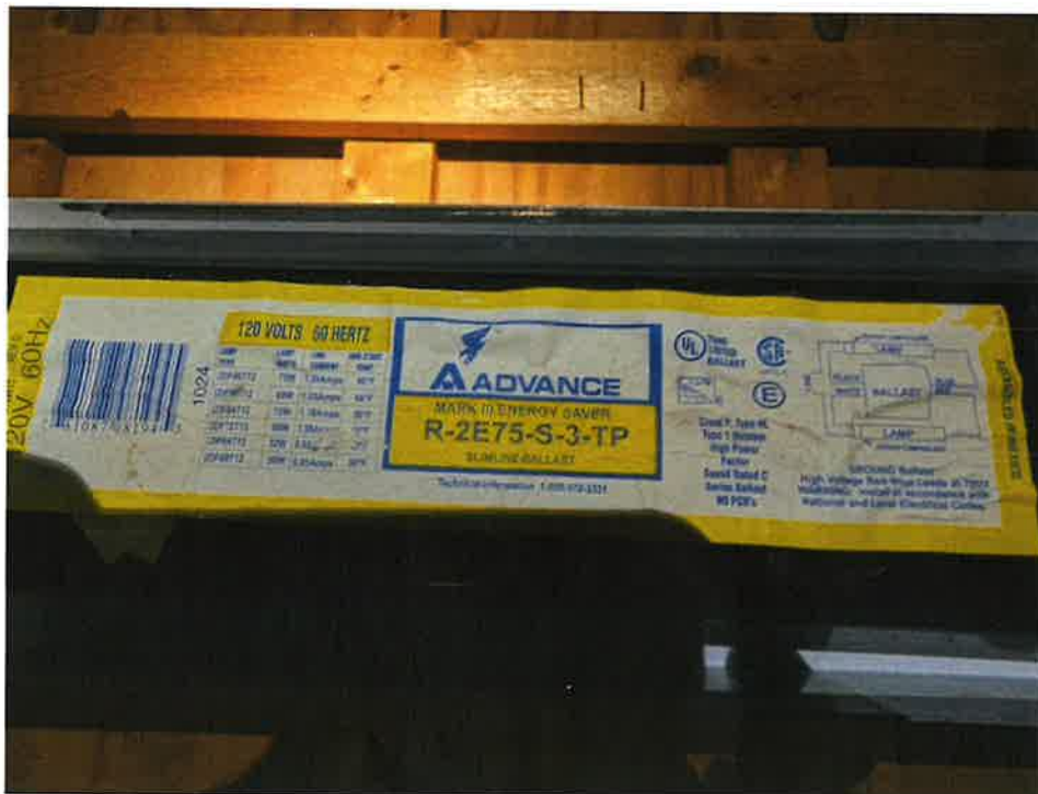
Photo 4: Non-PCB ballast in fluorescent fixture
