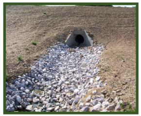
material. Stormwater that is transported through man-made conveyance systems at design capacity generally reaches a velocity that exceeds the ability of the receiving channel or area to resist erosion. To prevent scouring at stormwater outlets, a flow transition structure is required, which will absorb the initial impact of the flow and reduce the flow velocity to a level that will not erode the area of discharge.
