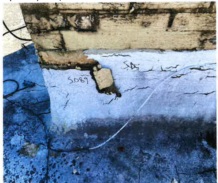
Picture 16. Sample S.089 flashing/caulking on chimney on roof (2% Chrysotile).
