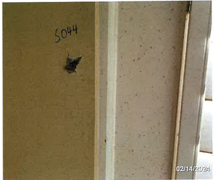
Picture 8. Sample S.044 in Bedroom #1 wall board (2% Chrysotile).
