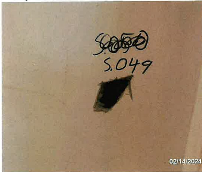
Picture 9. Sample S.049 Bedroom #1 Closet #1 wall board (2% Chrysotile).
