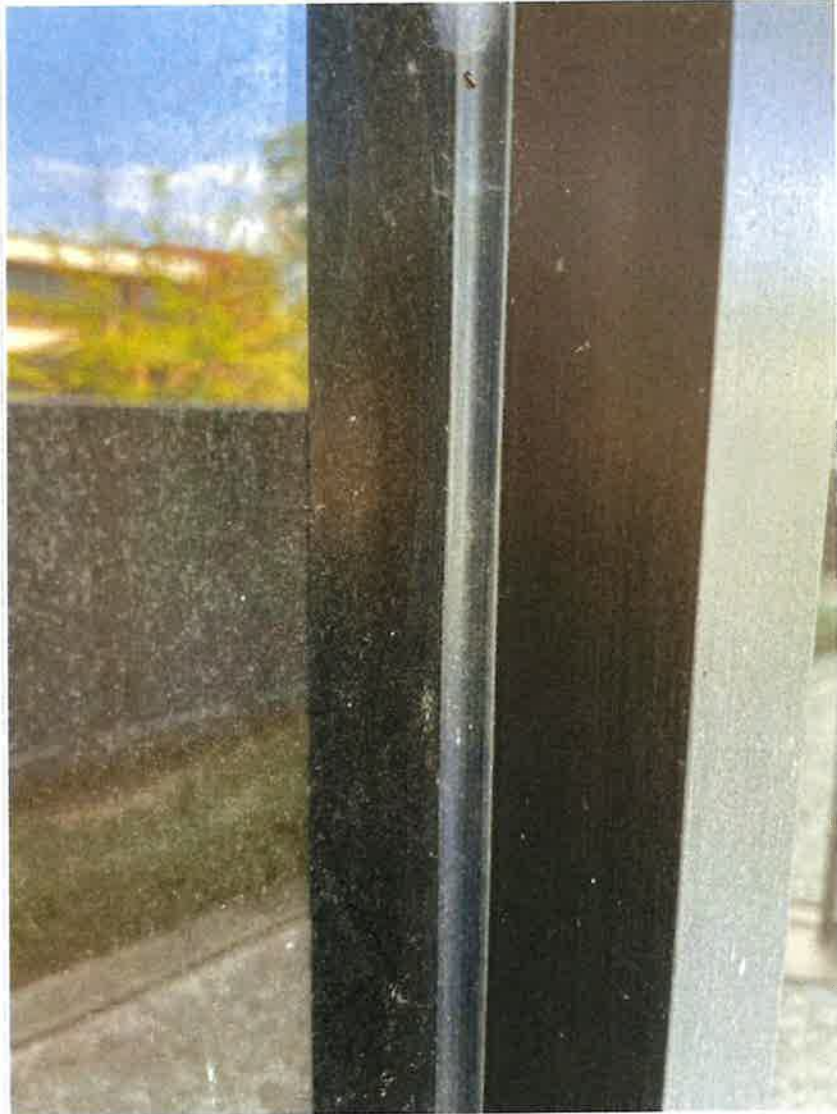
Exterior window glazing- rubber- non suspect
