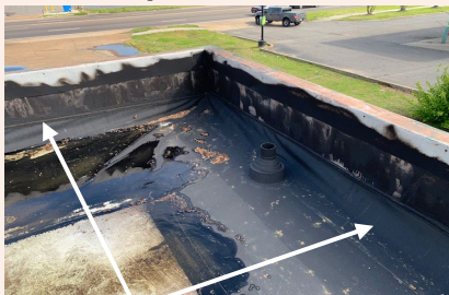
Parapet Wall MD-17
