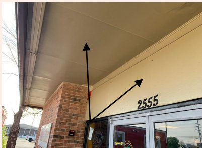
Front Transite Soffit
