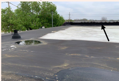
Parapet Wall MD-17
