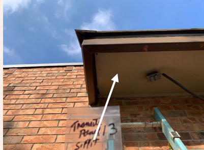
Side Transite Soffit
