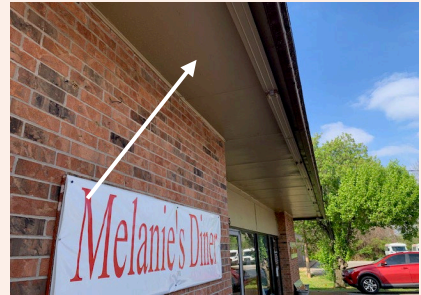
Front Transite Soffit
