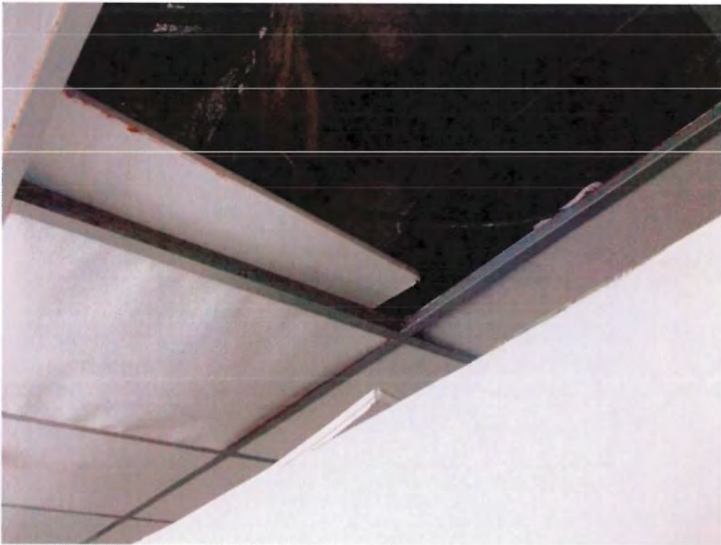
HSA 158-02: 2' x 2' Drywall Ceiling Panel. Sample B.
