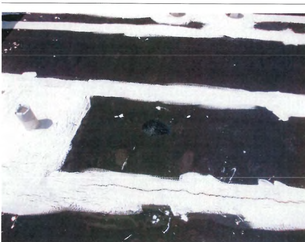
HSA 158-09: Roofing Materials. Sample A.
