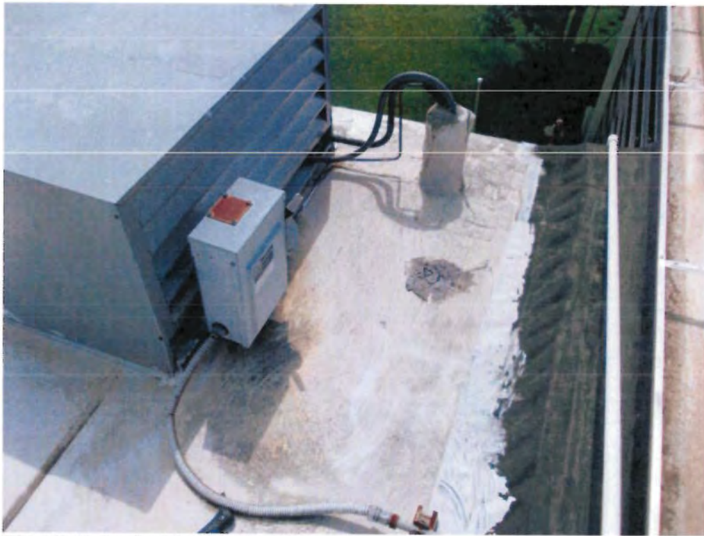
HSA 158-11: Roofing Materials. Sample B.
