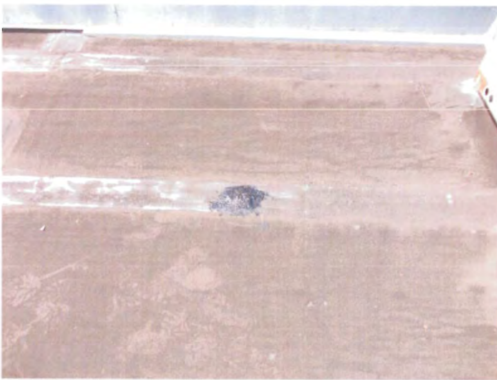
HSA 158-09: Roofing Materials. Sample B.
