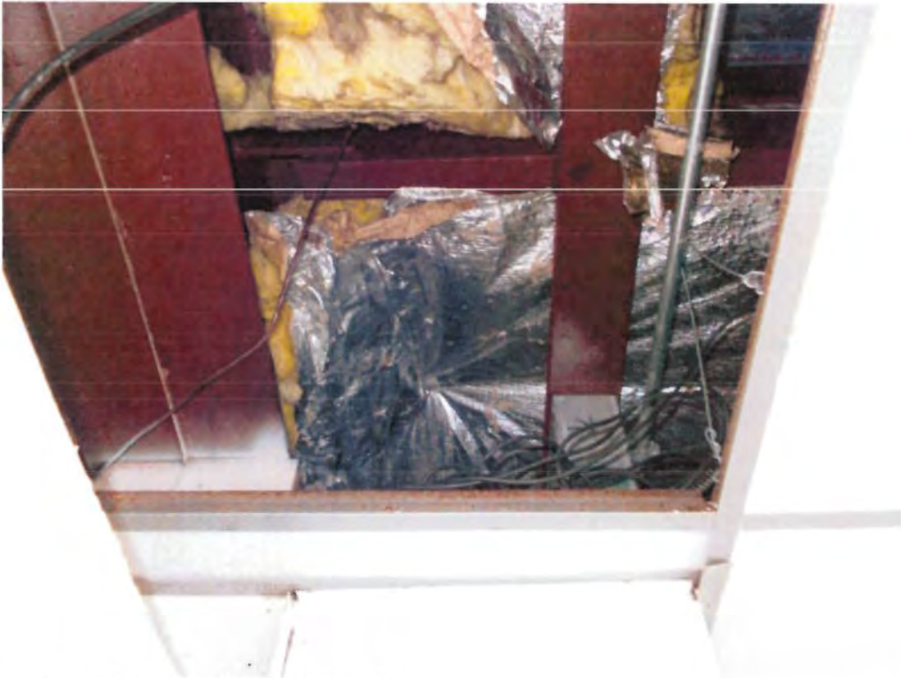
HSA 158-06: Roof Deck Insulation. Sample B.
