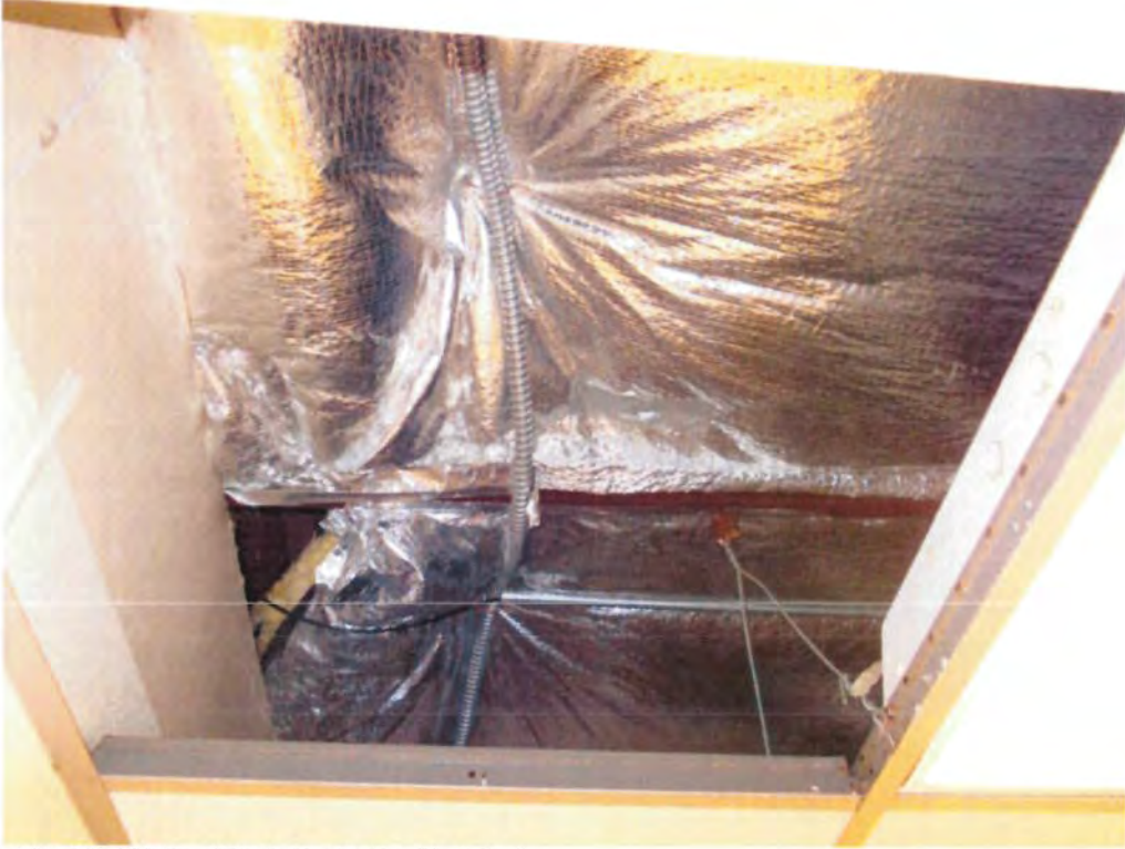
HSA 158-06: Roof Deck Insulation. Sample A.
