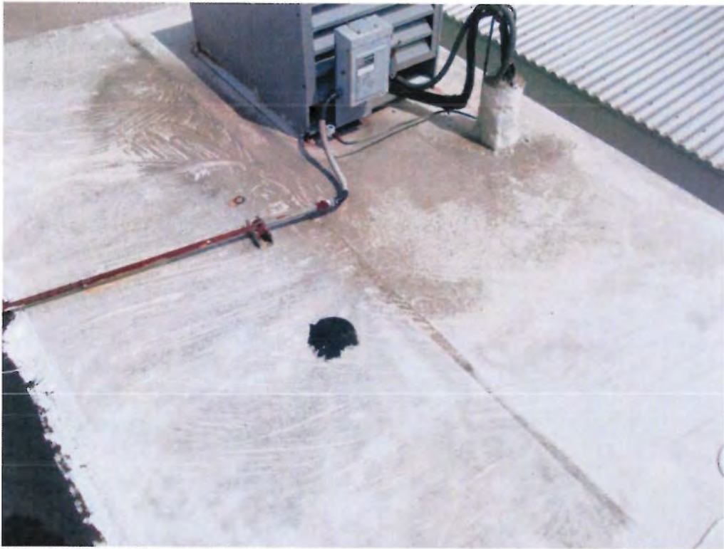
HSA 158-11: Roofing Materials. Sample A.
