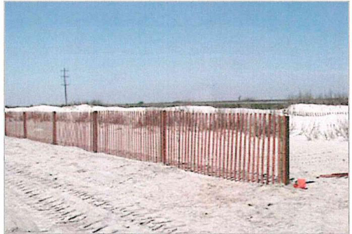
Figure 1 Sand Fence (<http://www.gulfmex.org/crp/7004/fence.jpg>)
