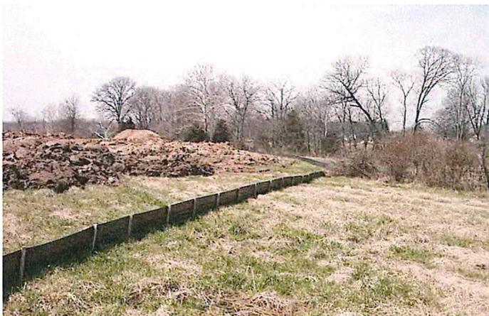
For Types A and B silt fence, place the bottom 12" of fabric in the 6" deep (minimum) trench, lapping toward the upslope side. For Type C fabric, place the bottom 6" in the 4" deep (minimum) trench lapping toward the upslope side.
