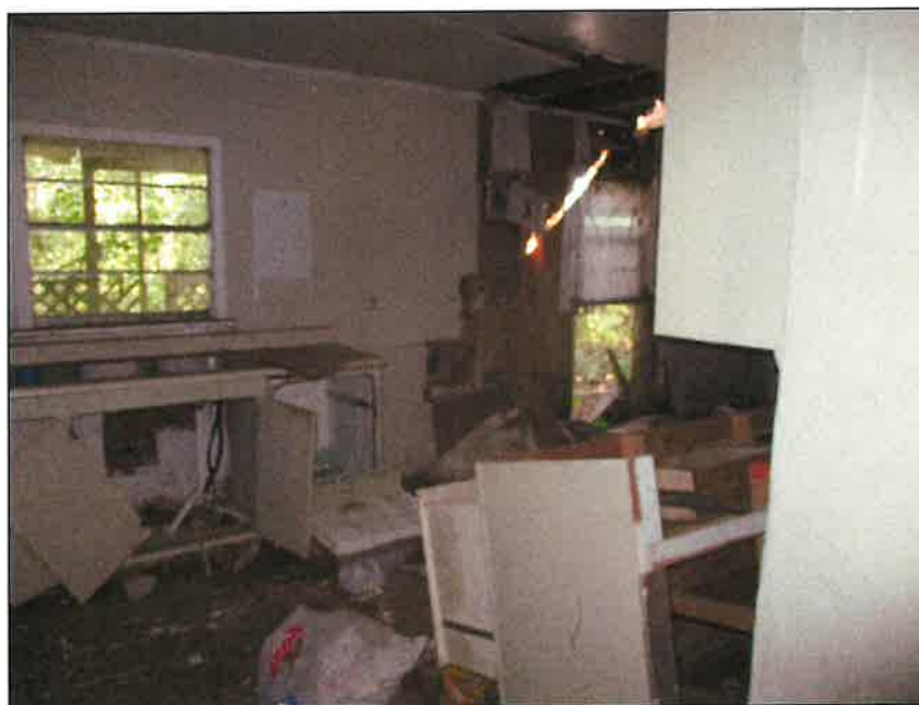
2 - View of the kitchen
