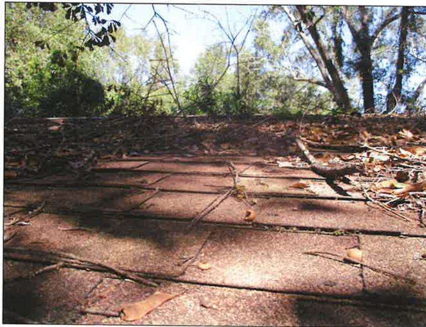
8 - View of the roof
