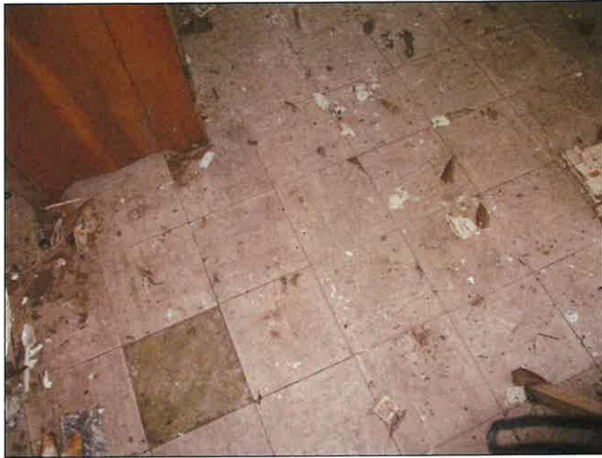
5 - View of the tan 9" x 9" floor tiles (ACM)
