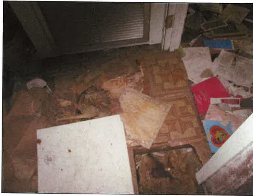
7 - View of the of brown linoleum
