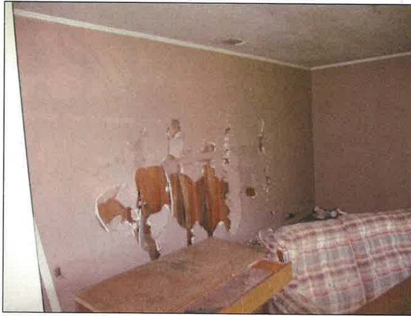
3 - View of the living room (ACM drywall)
