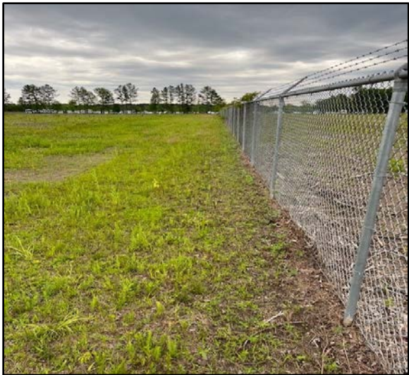
Photo 2 Fence North Side No Erosion Noted West View
