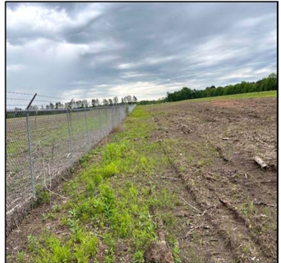
Photo 5 Fence Line South Side No Erosion Noted
