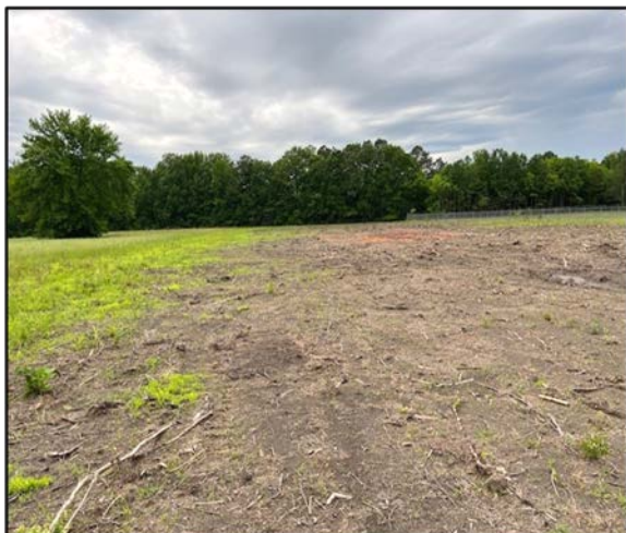
Photo 3 South Clearing Limits No Erosion Noted
