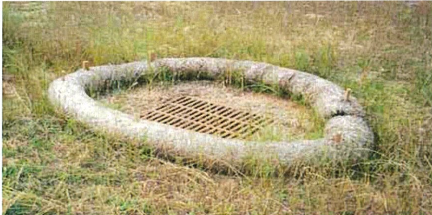
STORM DRAIN PROTECTION – wattle surrounding drain inlet
