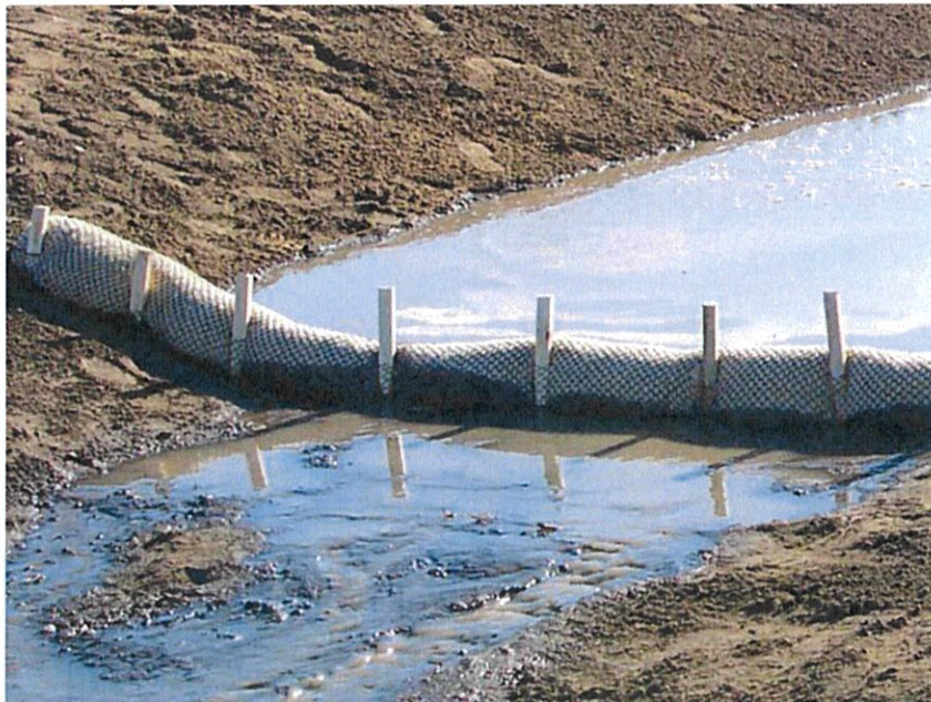
Wattle across storm drainage preventing downstream sediment transport
